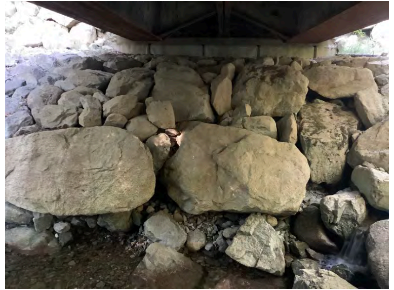
Right Bank Abutment when facing downstream
