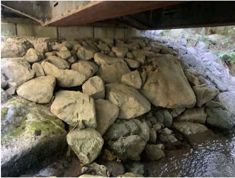
Left Bank Abutment when facing downstream
